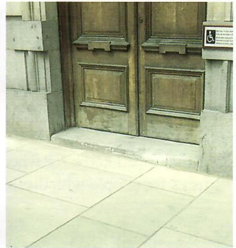
York stone paving at the Town Hall is well laid and provides a durable easily cleaned surface
