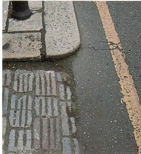
Victorian granite kerbs and access ramp
