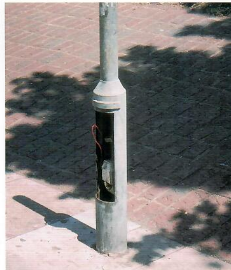
Redundant posts are removed
