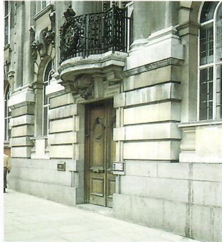
York stone paving at the Town Hall is well laid and provides a durable easily cleaned surface
