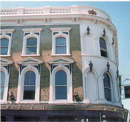
The former Atlantic PH, 1868, Coldharbour Ln.
