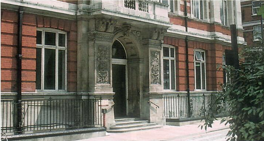
Renewed railings and sets in the road provide a more suitable setting for the Tate library
