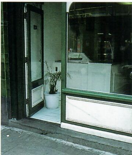
The door panel is as high as the stallriser
