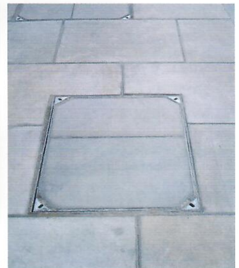
York stone or concrete paving is continued as a smooth or tactile surface across inspection covers
