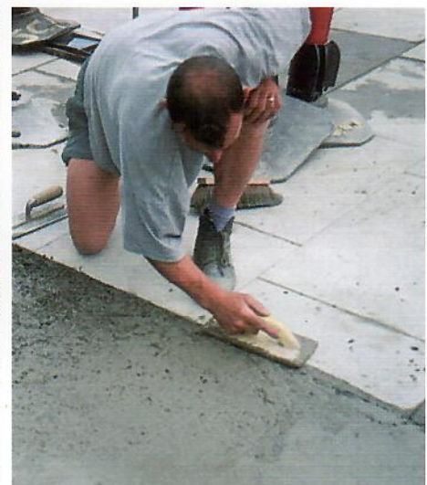
Added strength is needed to prevent damage near kerbs. Care is needed in finishing
