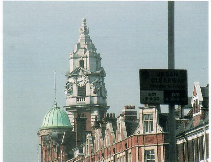
The Town Hall tower is seen in the background of many views of Brixton
