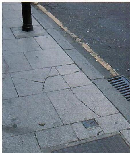
Added strength is needed to prevent damage near kerbs. Care is needed in finishing
