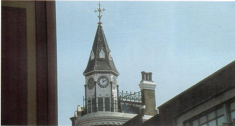
Brixton's buildings have many fine landmark towers, turrets, domes and spires
