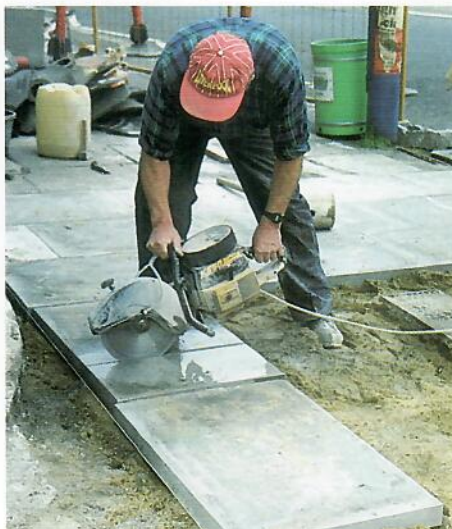
Ordinary concrete paving in Brixton is designed, cut and laid with the same care that is given elsewhere to expensive York stone paving
