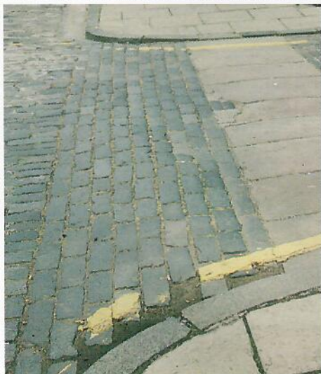
Yellow lines are difficult to maintain; here at a smooth stone crossing on a sett carriageway, at an enhancement scheme and at a dropped kerb
