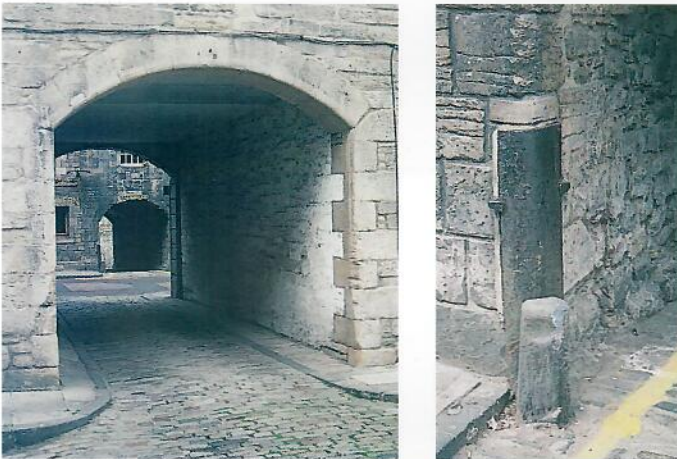
Across the High Street the far arch is protected by a stone bollard
