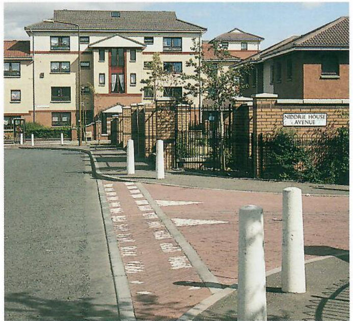
Traffic calming at an internal junction. A consistent approach
