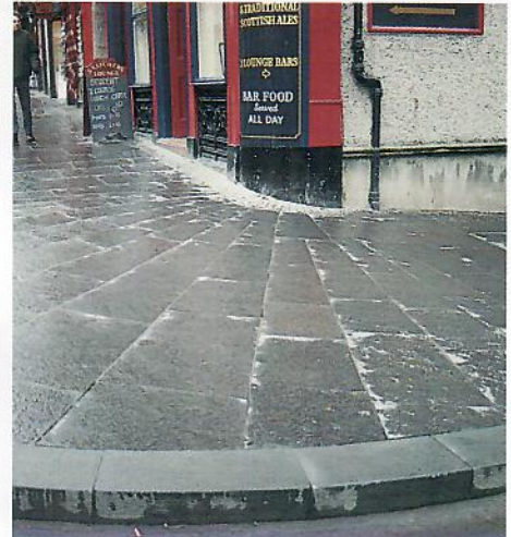
Radiused paving slabs in the High Street
