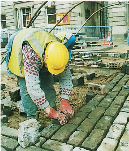
Laying setts across a carriageway
