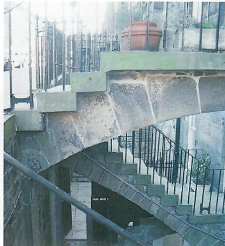
Typical flying buttress arches supporting steps Steps overlap the one below
