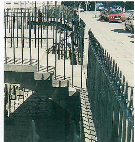
Typical flying buttress arches supporting steps Steps overlap the one below
