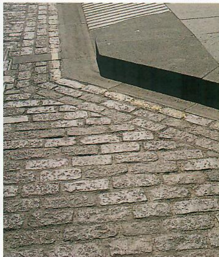
Three rows of setts parallel to stone channel
