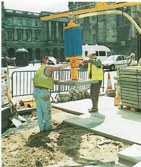
Natural stone slabs being lifted by machine
