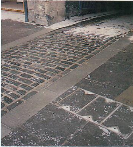
Setts where vehicles cross the pavement
