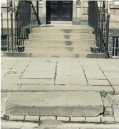
The layout of the pavement slabs at Charlotte Square is centred on lines from the front doors of the houses to the mounting stones at the kerb
