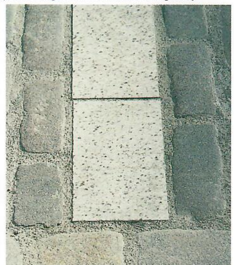
White lines to mark parking bays in sett carriageways can be formed of light grey stone setts
