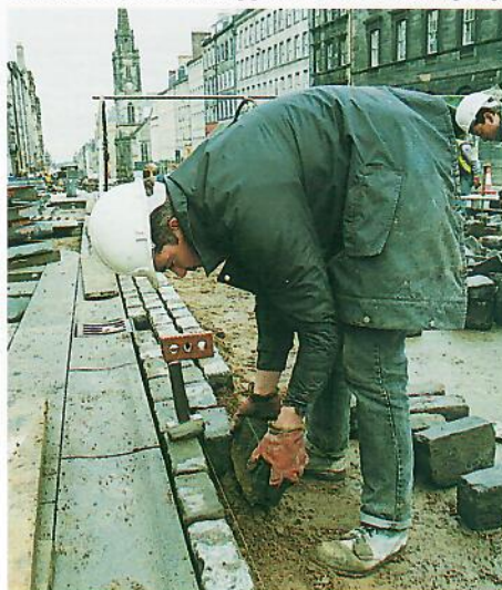
Laying setts against drainage channel
