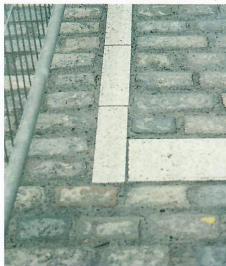
White lines to mark parking bays in sett carriageways can be formed of light grey stone setts
