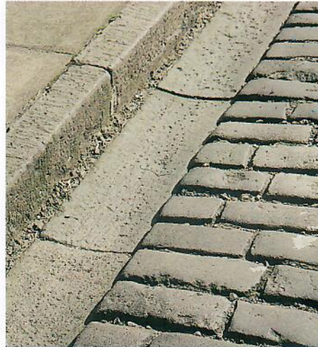
Typical setts, kerb and drainage channel
