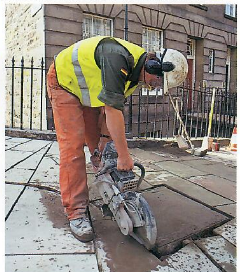
Cutting concrete slabs at an inspection cover
