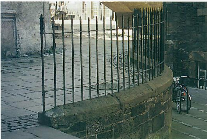
Sett drainage channel, stone retaining walls, iron railings in a close
