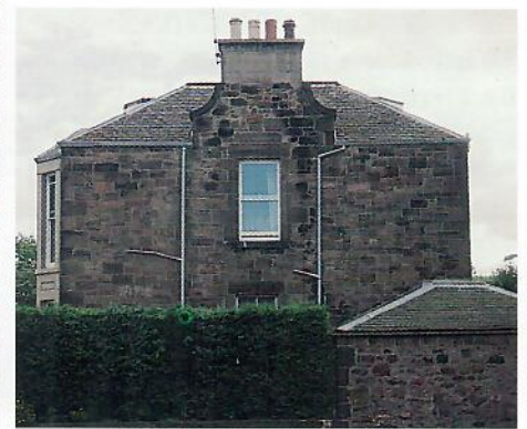
House at the corner of St Catherine's Place
