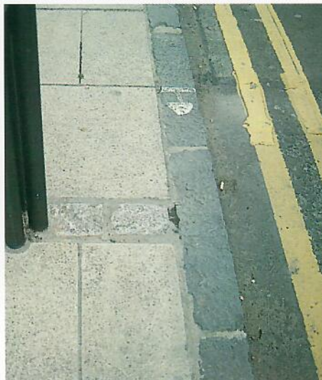
Yellow lines are difficult to maintain; here at a smooth stone crossing on a sett carriageway, at an enhancement scheme and at a dropped kerb
