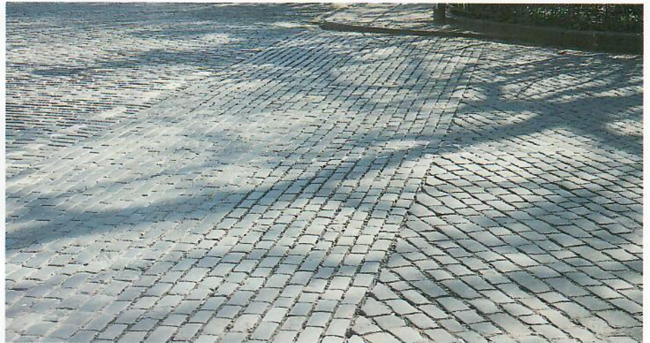
Places where pedestrians cross the road at junctions are often marked by different sized setts
