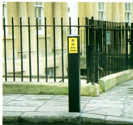
New shape sign fixed to a bollard
