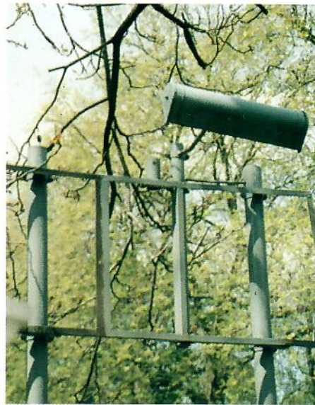
Redundant sign frames
