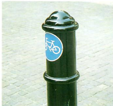
Unauthorised curved sign on a bollard
