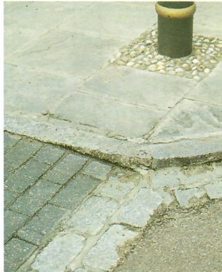
Paving at kerb
