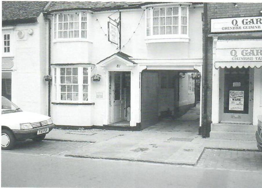
Cross-over with parking bays at Buntingford
