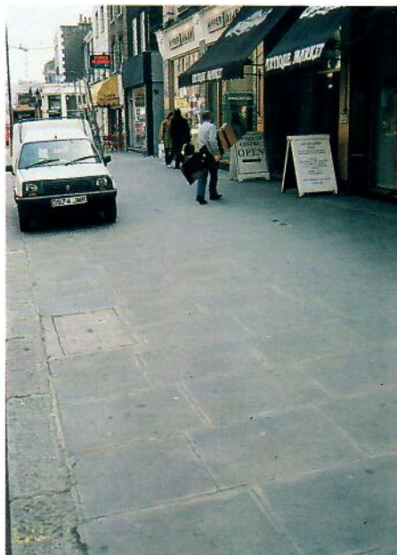
Large concrete slab paving at Chelsea
