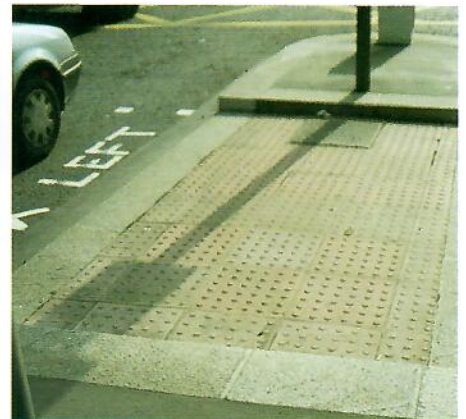
Tactile surface at pedestrian refuge
