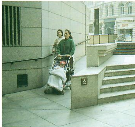
Ramp at steps
