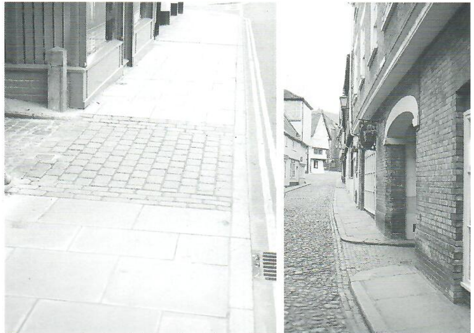
The cross-over treatment at Norwich retains much of the character of a traditional access
