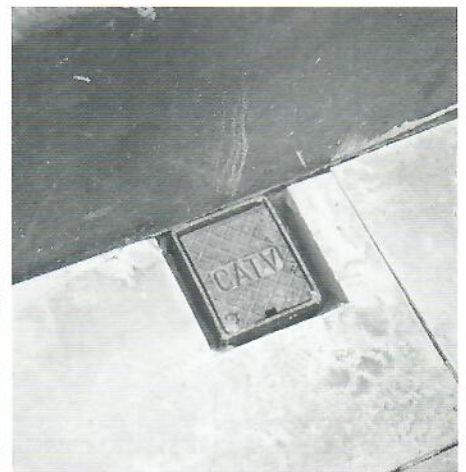
Accurate cutting at inspection covers
