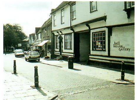
The carriageway is raised and narrowed
