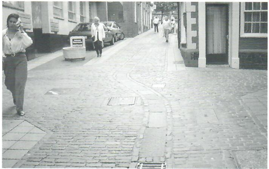
A granite central drainage channel follows the curve of the street, Norwich
