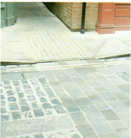
A smooth passage across granite setts
