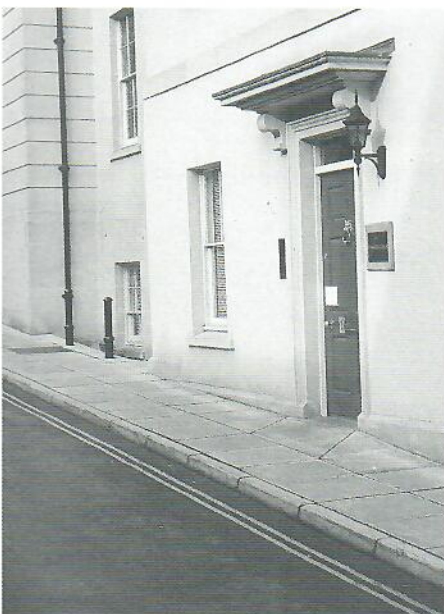
50mm lines. DoT authorisation not needed
