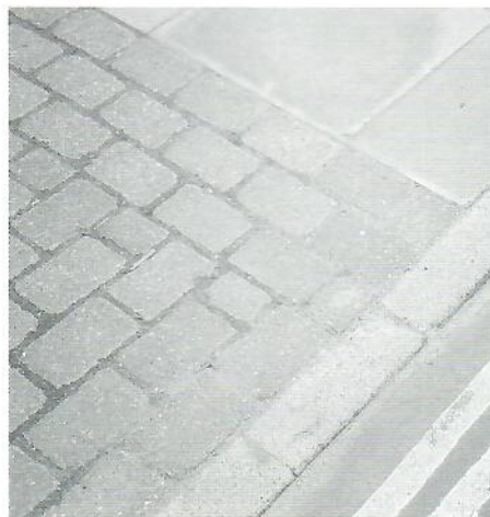
Slab edges have been strengthened
