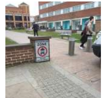
7.07 Neatly fixed zone signs
