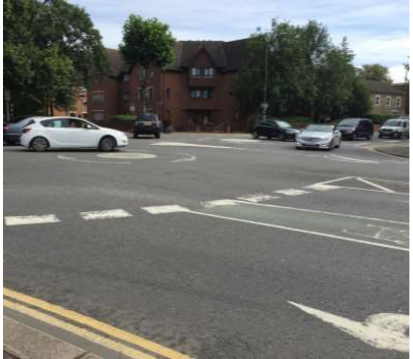
9.11 Drivers are quite familiar with and able to cope safely at double mini-roundabouts such as at Bromham Road, A280, Bedford
