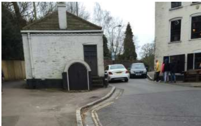
3.10 The seemingly dangerous pinch point where the road changes direction and level has a good safety record: one slight accident in 10 years (source Crashmap). Spaniards Toll Gate, Hampstead, London
