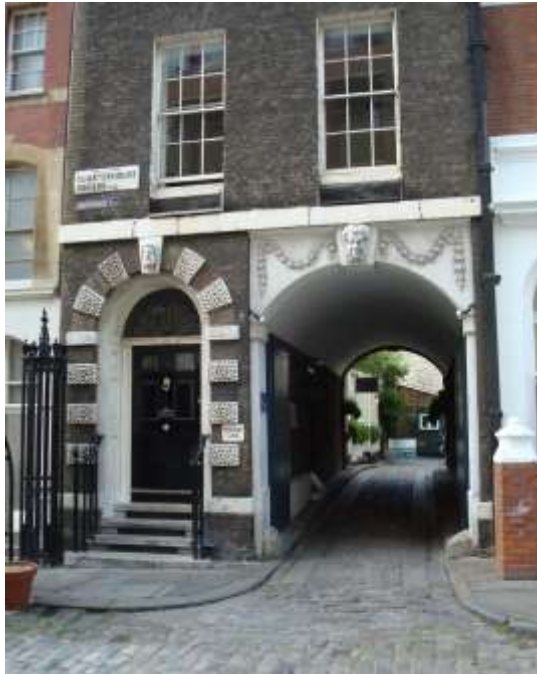
1.08 Traditional building with its prestige entrance for people directly from the street and a vehicle access at the side
