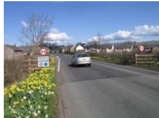
2.18 Clifton, Cumbria. White line removed on A6
