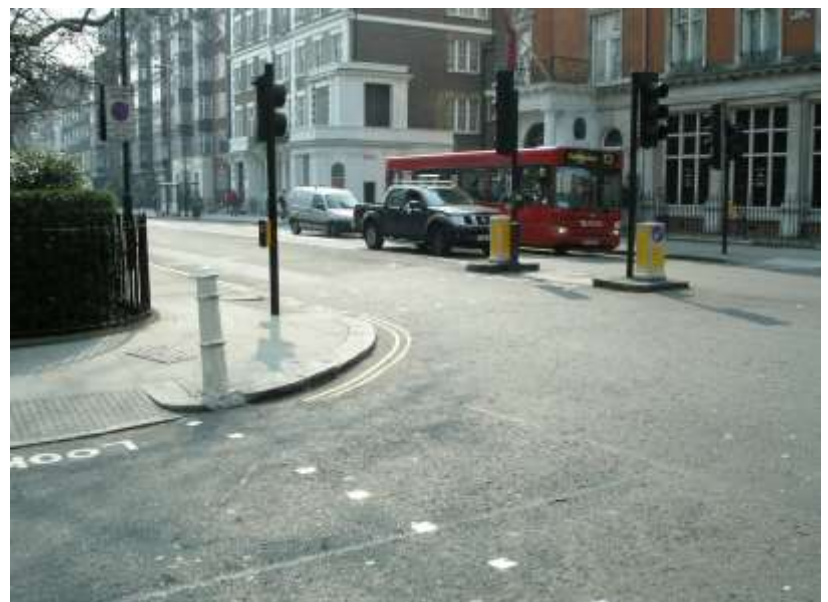
2.27 A tight kerb radius at Sloane Street, London, is typical of the Georgian and Victorian street layouts in many historic town centres
