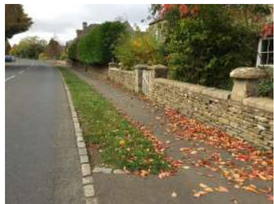
11.06 New subtle grass verges narrowed a section of the road, fitted seamlessly into the appearance of the village and helped reduce traffic speed
