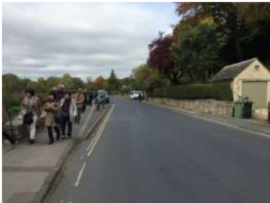
11.07 Parked cars that effectively narrow the road and the removal of road centre white lines reduced traffic speed
