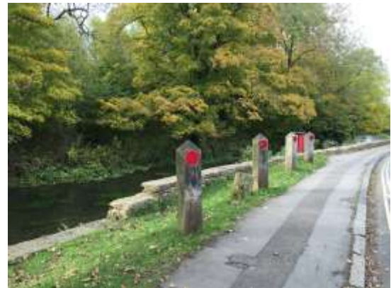
11.05 Ugly chevron warning signs were replaced with rural-style wooden posts with reflective discs
