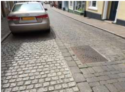
4.09 Distinctive road surface indicates parking places. Bury St Edmunds, Suffolk
