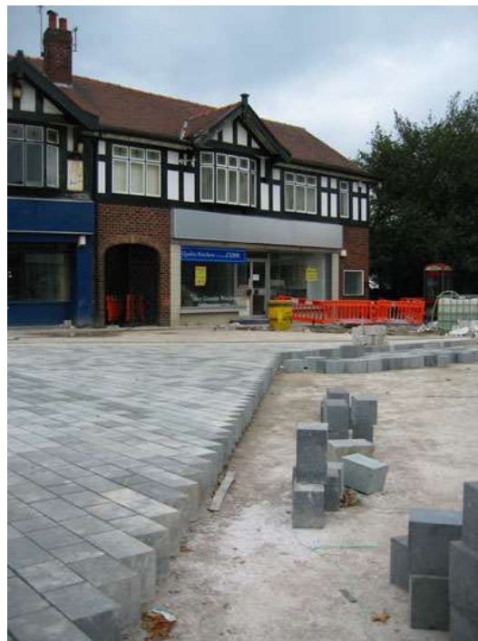
9.04 The project under construction in 2010
