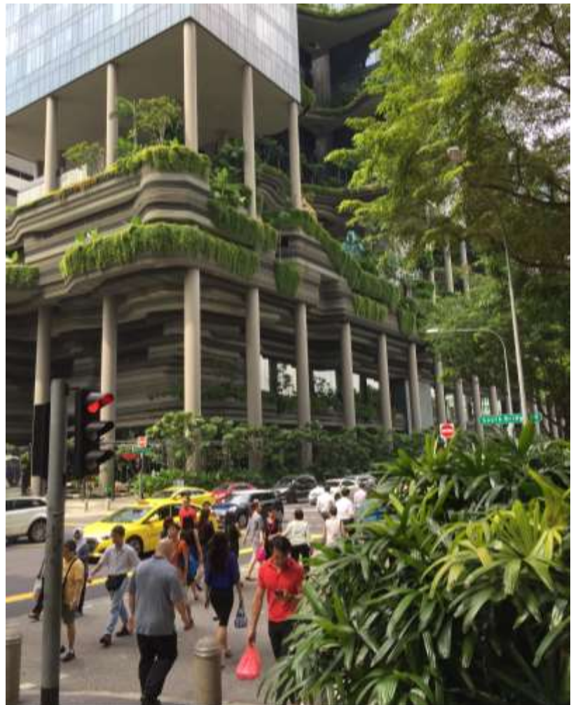
4.16 Co-ordinated greening of roads and buildings. Singapore
