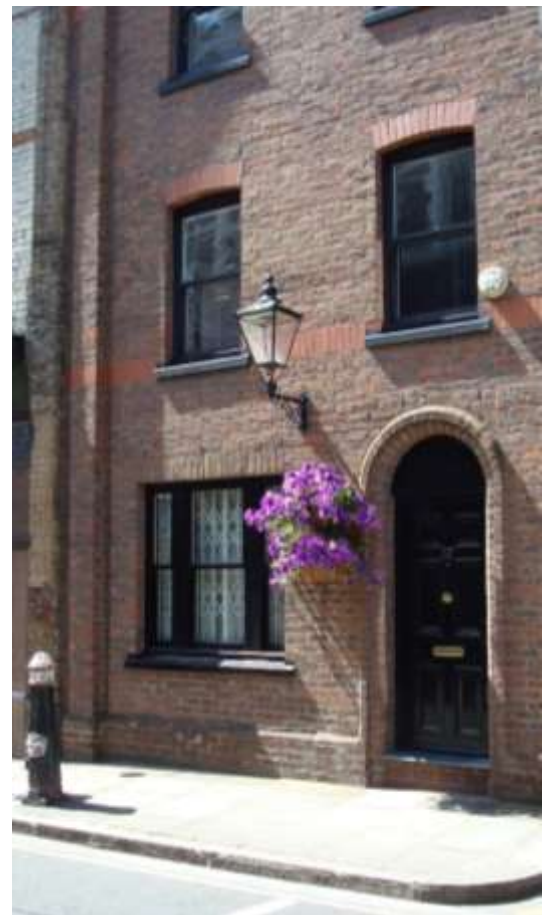
4.17 Public street lighting fixed neatly to buildings. Middle Street, City of London
