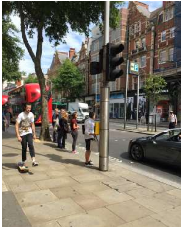
8.07 A simplified traffic light (signal) fixing is combined on a single column with street lighting
