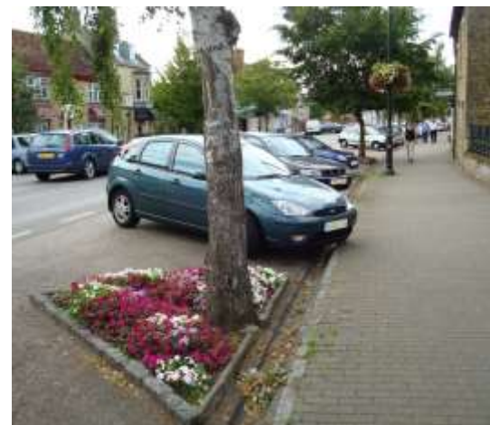
2.20 Right angled parking calms traffic on A509
