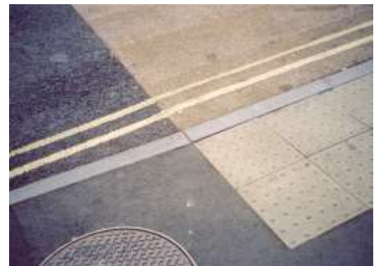
4.13 Tidily installed tactile paving and the neater narrow version of yellow lines
