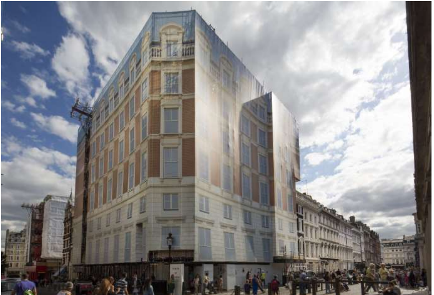
4.18 Building construction works concealed behind a temporary trompe-l'oeil
