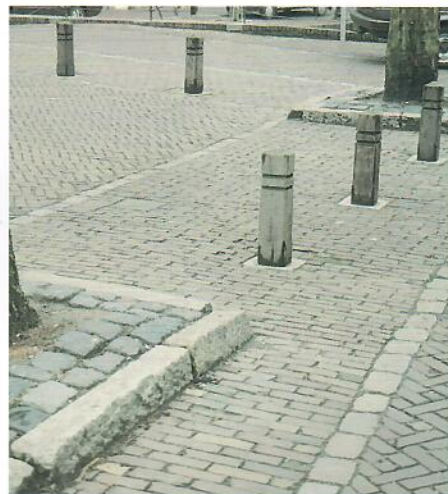
Surface for vehicles indicated by a subtle texture change and equally spaced bollards
