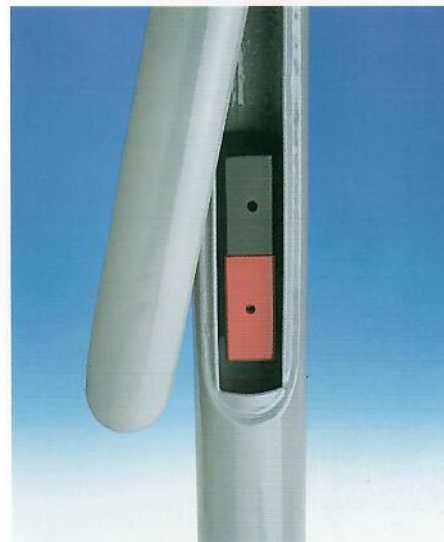
Electrical supply is within a narrow post
