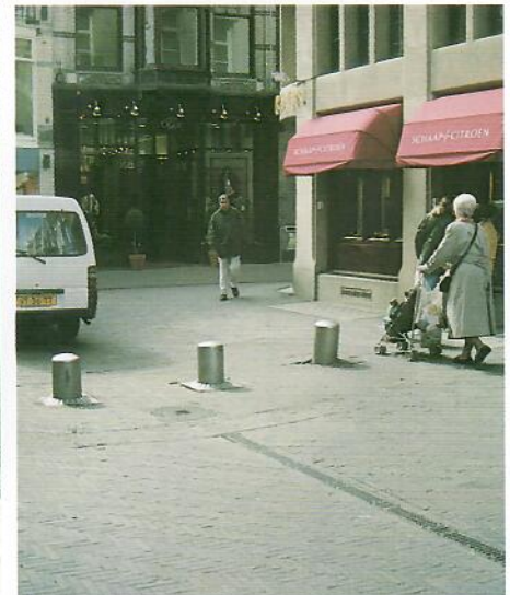
Bollards lower into ground at the zone edge
