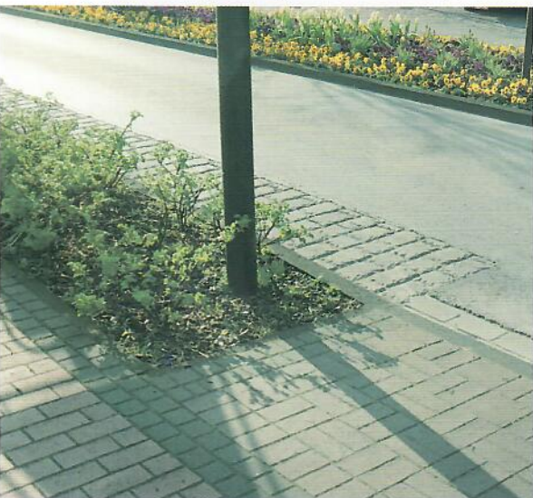
Carriageway surface texture to encourage safe driving is co-ordinated with footway crossing
