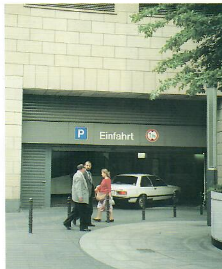
Entrance to an urban car park, Dusseldorf
