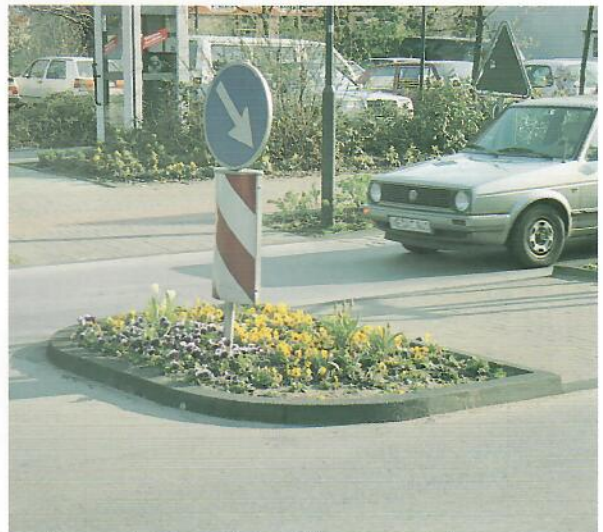
The road is narrowed where pedestrians need to cross the road from a car park
