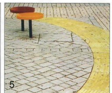
2 No tactile surface at a side road dropped kerb; 3 Unnecessary tactile surfaces at a locked private gateway; 4 One of the confusing official advisory diagrams. This conglomeration of surfaces becomes even more ludicrous when applied to real streets; 5 A tactile surface used purely as decoration
