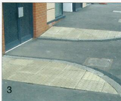
2 No tactile surface at a side road dropped kerb; 3 Unnecessary tactile surfaces at a locked private gateway; 4 One of the confusing official advisory diagrams. This conglomeration of surfaces becomes even more ludicrous when applied to real streets; 5 A tactile surface used purely as decoration
