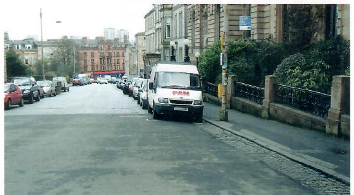
Yellow lining can look garish ( top, left ) and is difficult to apply to traditional materials ( top right ). Neatly-applied 50mm primrose-coloured lines can make a difference ( middle ) and a new road-marking regime in a restricted parking zone ( bottom )
