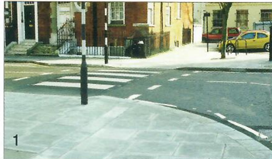
1 Blister paving sensibly applied at a zebra crossing. Tonal differentiation is where it is needed, at the dropped kerb;
