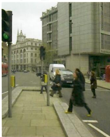
Pelican crossing without guardrail
