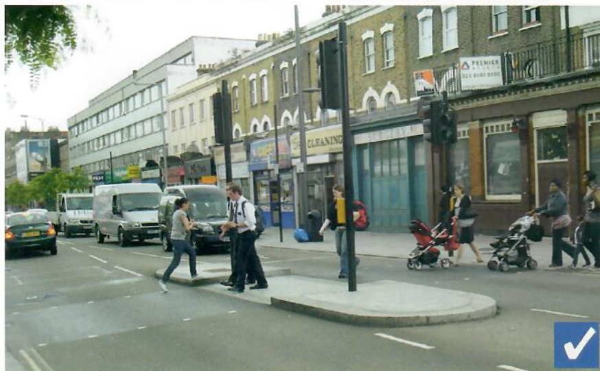
Signal controlled crossing without a keep left sign
