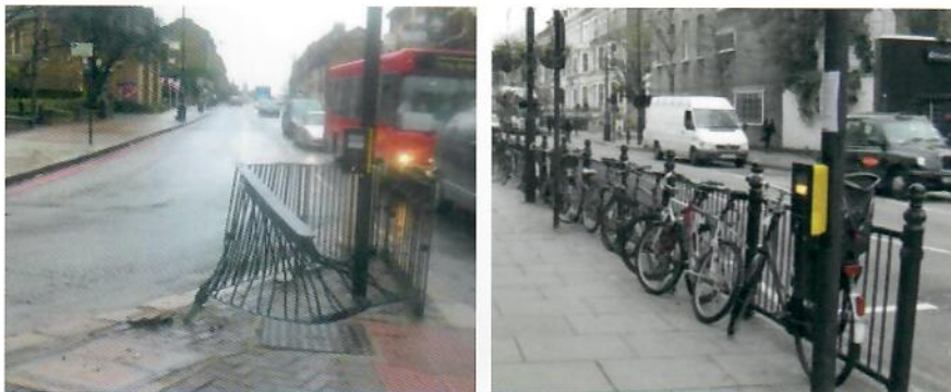
Guardrailing is not intended to protect pedestrians but may provide parking for cycles
