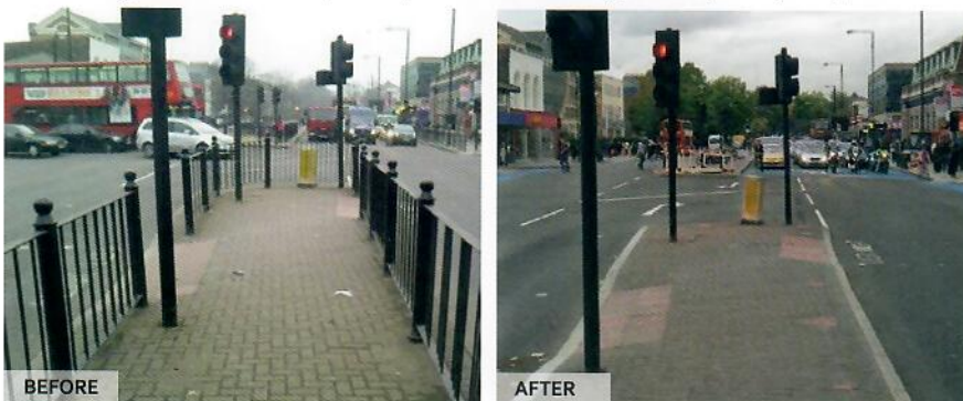
At many of the TfL crossings, guardrailing was removed without any other associated works
