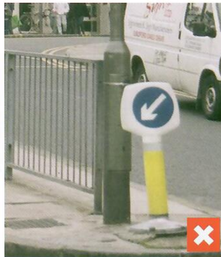
Unnecessary sign and guardrailing
