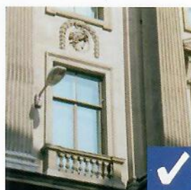
Street lights on buildings
