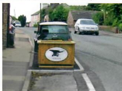
Build-outs with planters bearing a white motif Width of road at build-out: 6.0m No centre of road white line
