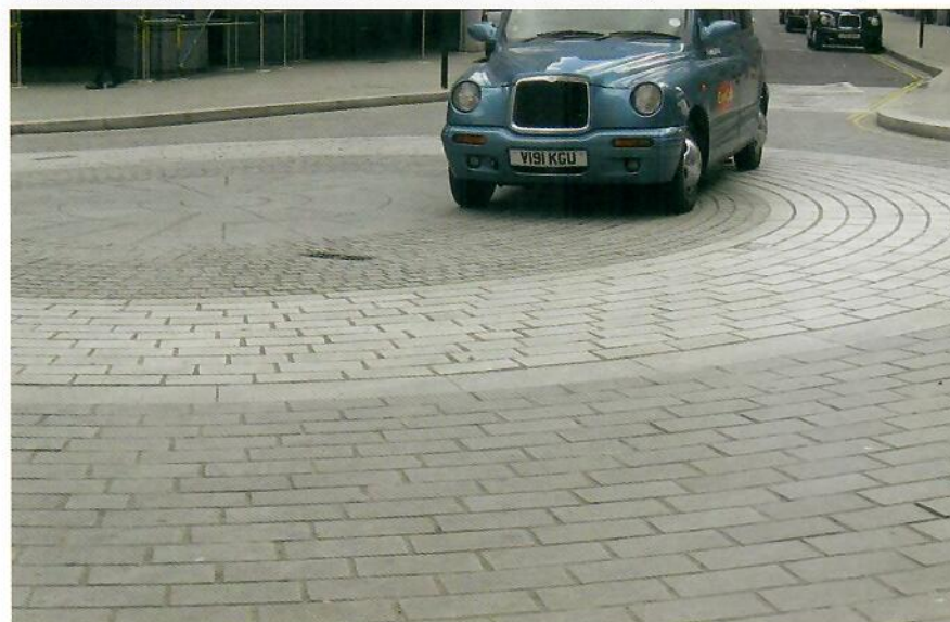
Surface materials at an uncontrolled junction with courtesy crossing help drivers to negotiate
